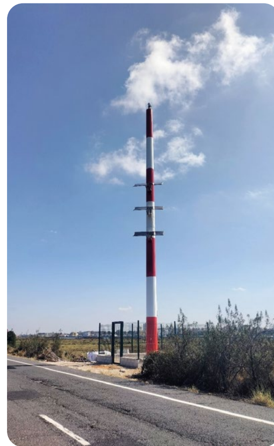
Camera installed on the dyke road.
