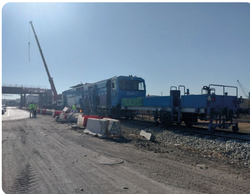
Rehabilitation of track 2S2 (during works).
