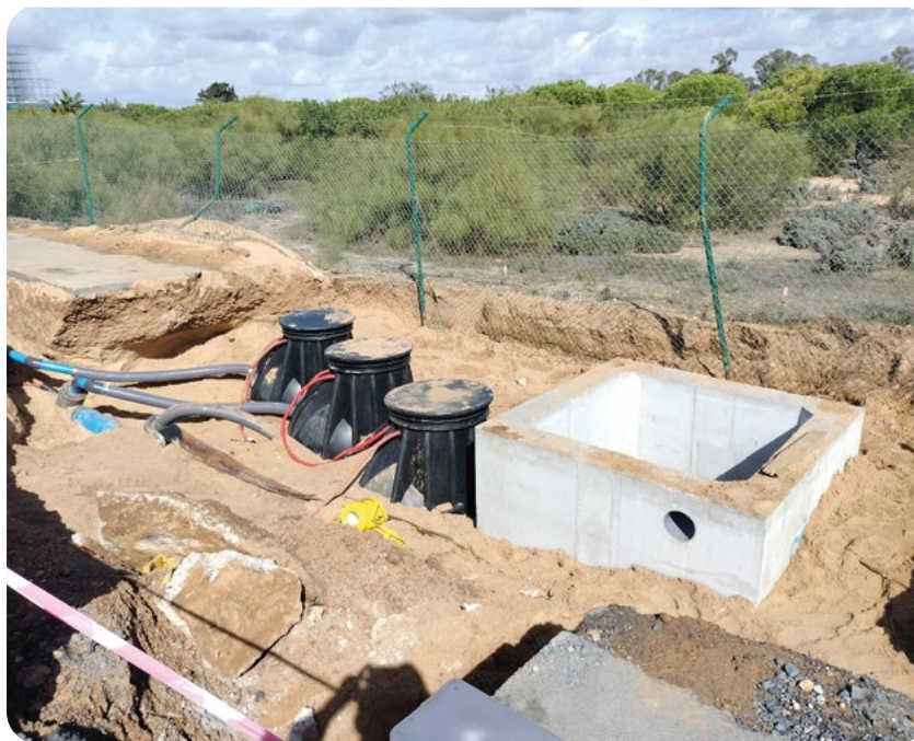
South quay drainage connection (during works).
