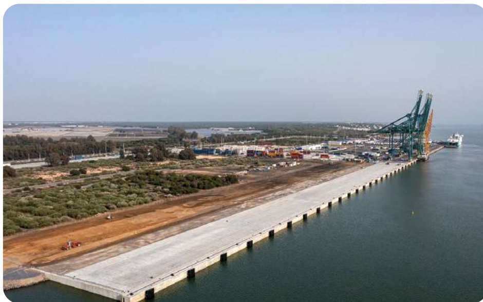
North Extension of the South Wharf (after completion of works)
