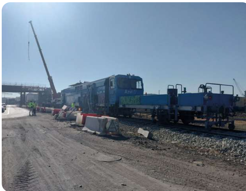
Rehabilitation of track 2S2 (during works).
