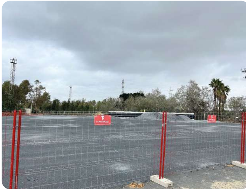
Extension of Punta del Sebo car park (during works).
