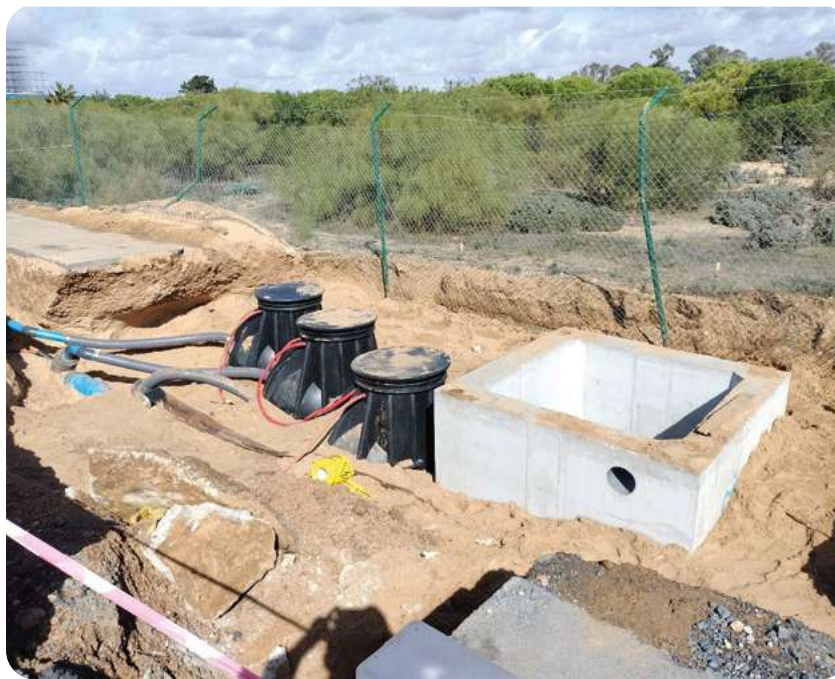
South quay drainage connection (during works).
