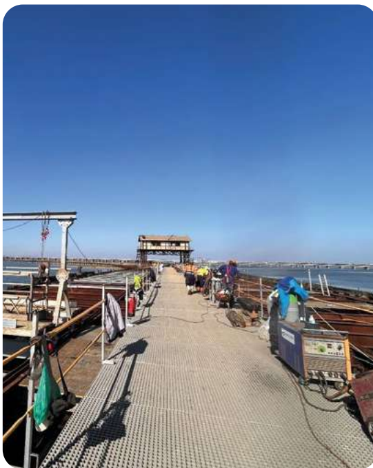
Rehabilitation of the Tharsis Wharf (during the works).
