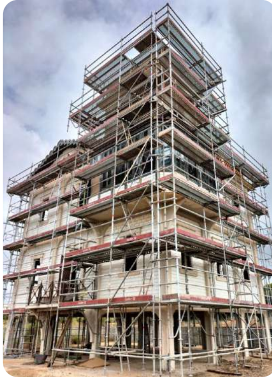
Refurbishment of Casa del Vigía (during the works).
