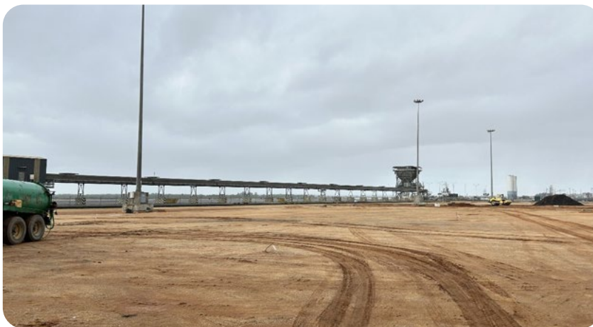
Expansion of the pavement of the Minerals Wharf (during works).
