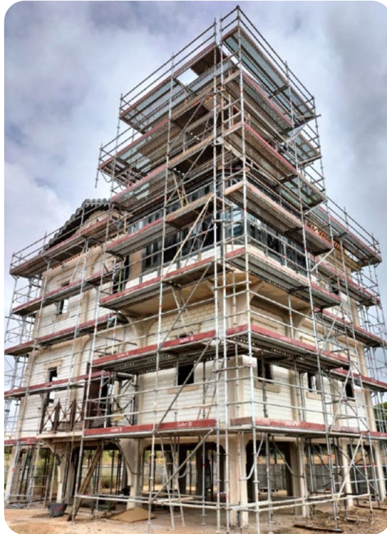
Refurbishment of Casa del Vigía (during the works).
