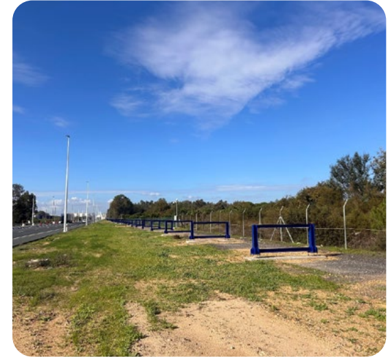
Rack for cold pipeline (during construction works).
