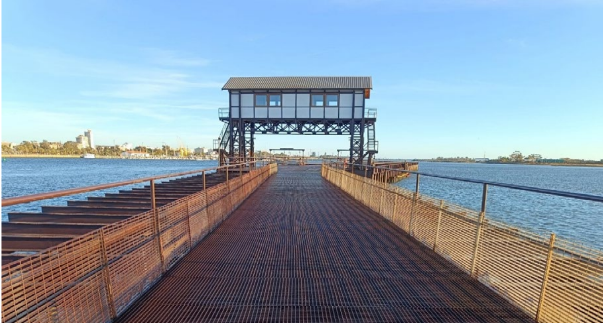
Tharsis Quay Restoration (completion of works).
