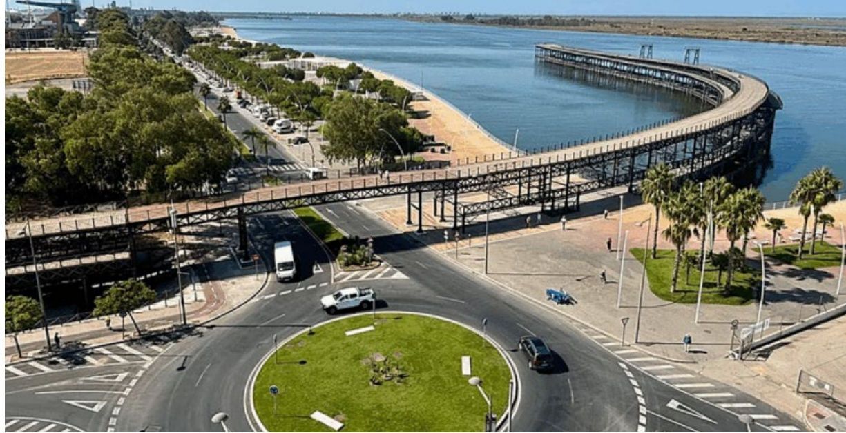
Riotinto Wharf Junction (completion of works).
