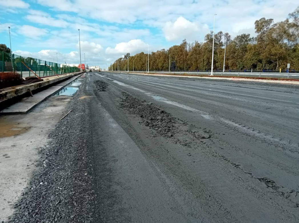
Railway terminal expansion (during construction).
