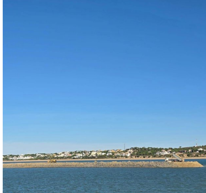
Site No. 4 Phase 2 (during construction).
