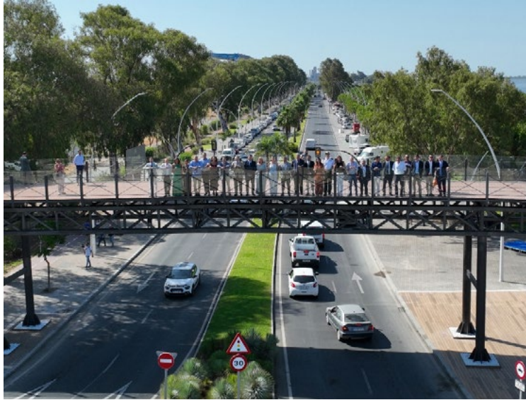
Opening of the Muelle del Tinto link.
