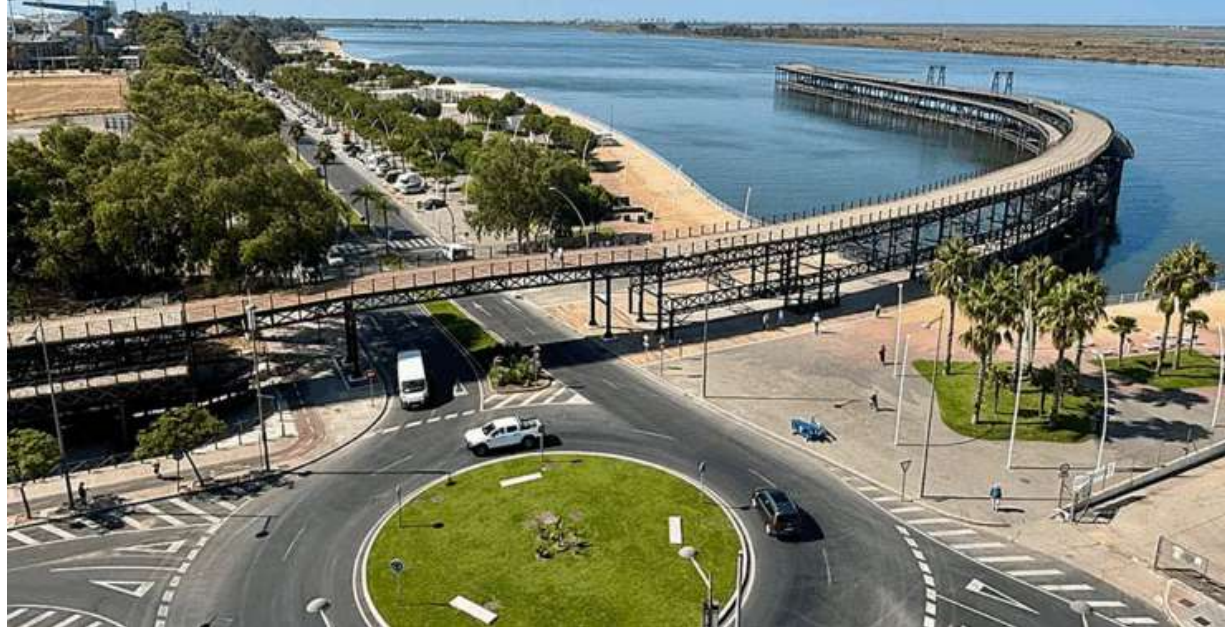
Riotinto Wharf Junction (completion of works).
