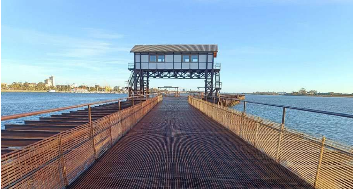
Tharsis Quay Restoration (completion of works).
