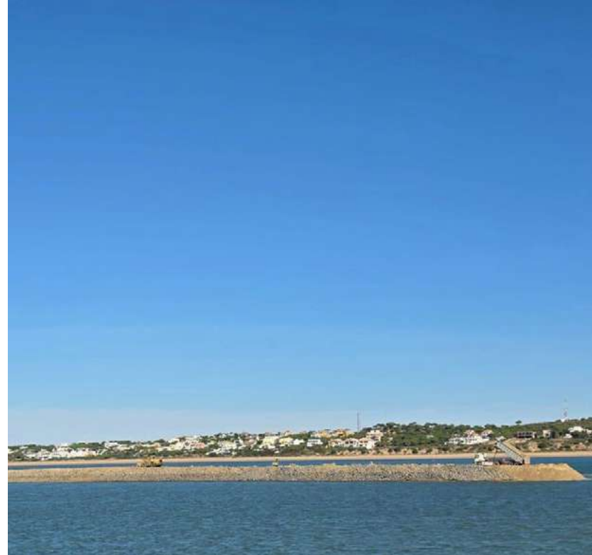
Site No. 4 Phase 2 (during construction).
