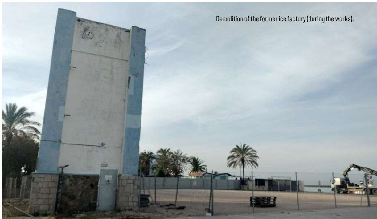
Cold pipeline rack (during construction),
