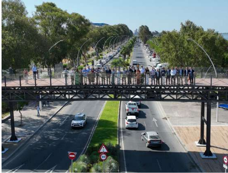
Opening of the Muelle del Tinto link.
